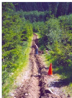
Figure 21: Burying the initial water line.
