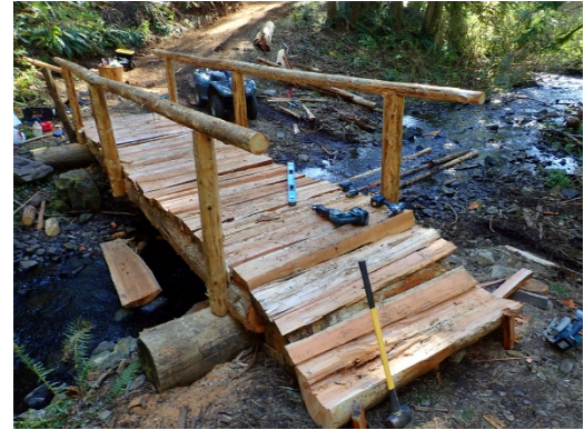
Figure 17: Finishing up the second footbridge.
