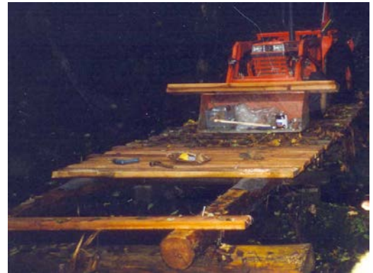
Figure 15: Building Earl's footbridge.
